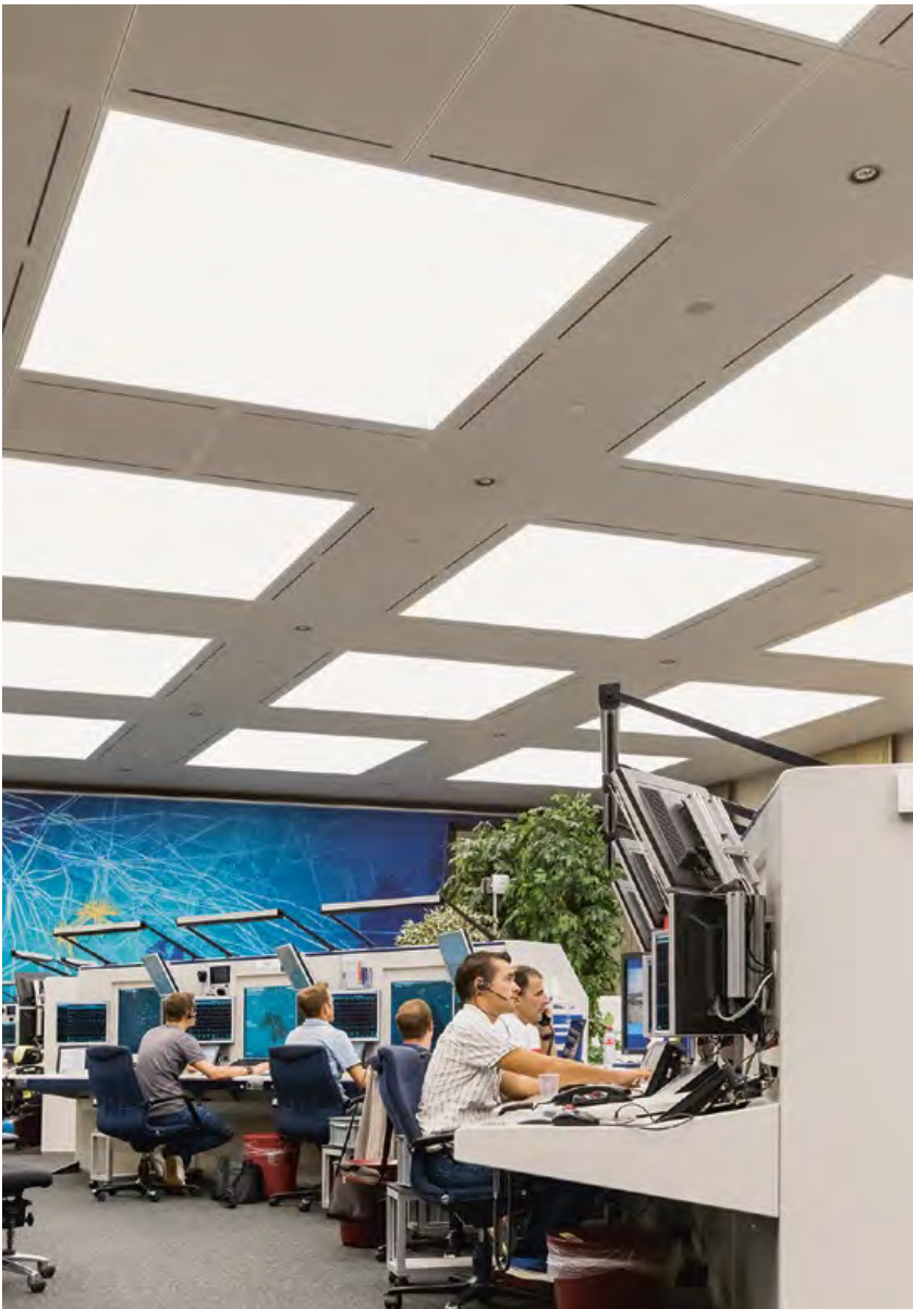
Ceiling lighting in the Wangen control center
