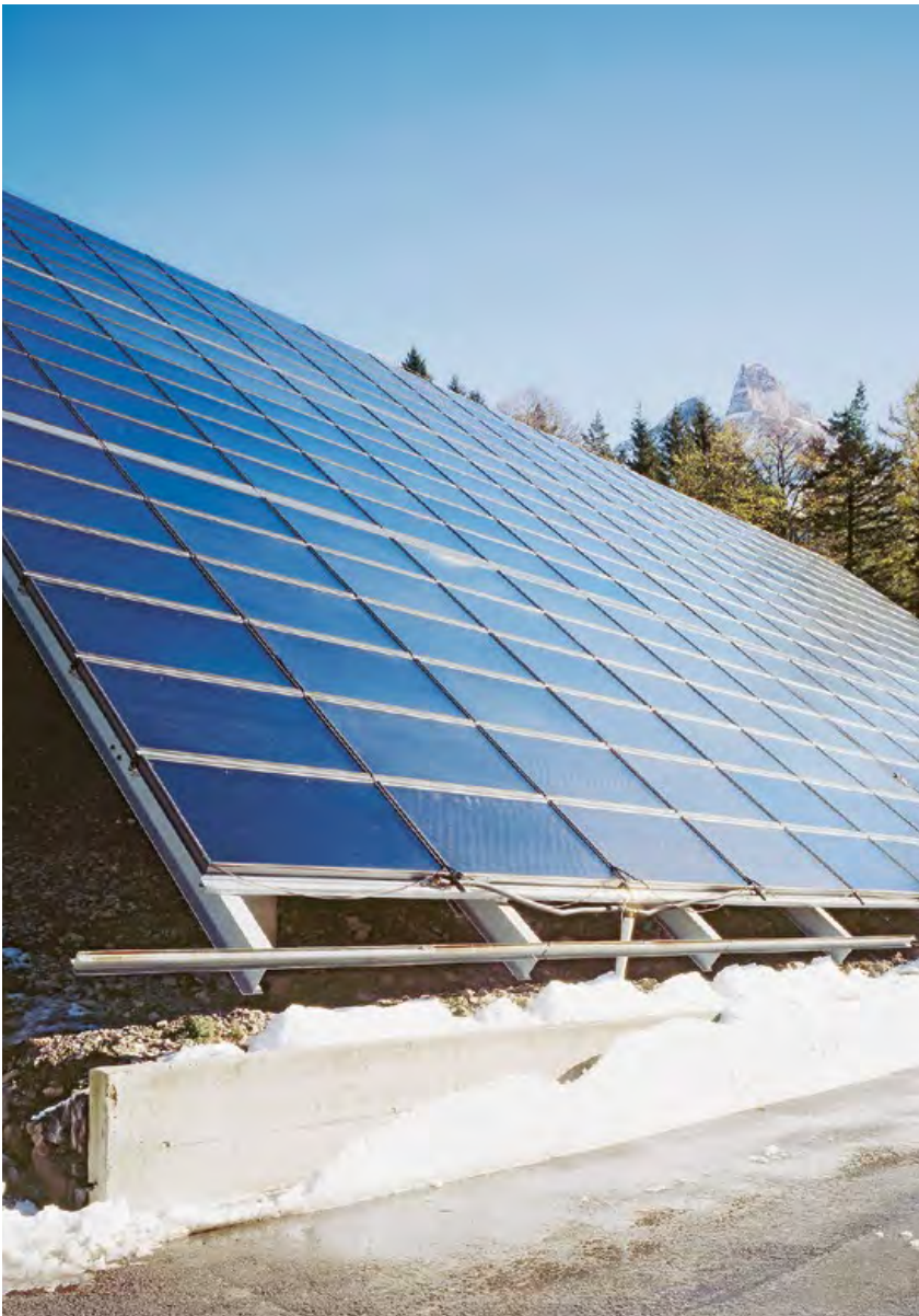
Solar thermal collectors installation at Dailly barracks, Vaud
